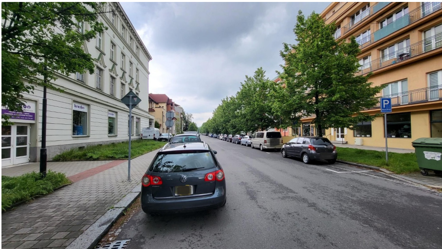
Figure 8 Eye-level view of Vítězná Street, illustrating active frontage, main-tained greenery, and usable sidewalks alongside traffic exposure and limited crossing opportunities. Source: Vítězná street, own picture
